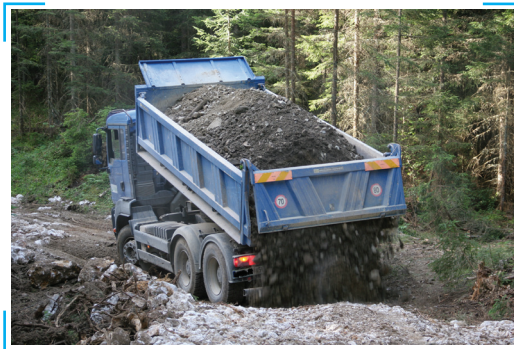
Picture 25: Trucks are used to transport and spread the material (Photo: Juri Beguš)
