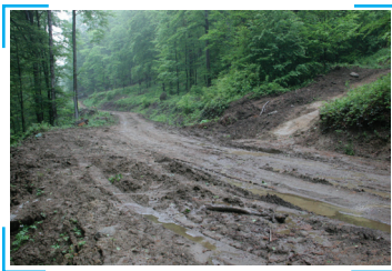
Picture 28: Consequences after forestry operations in the conjunction of forest road and skid trail (Photo: Juri Beguš)
