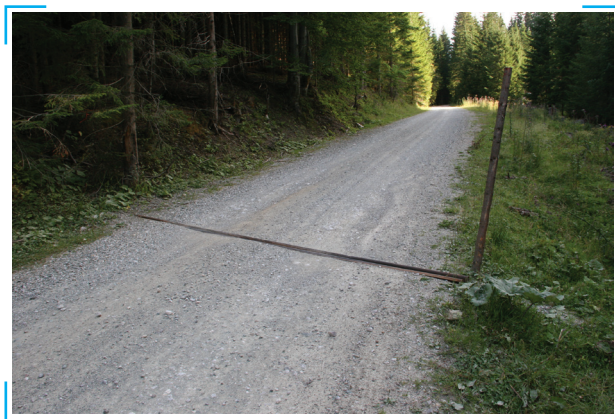
Picture 17: Cross ditch (Photo: Juri Beguš)
