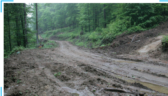
Picture 2: When forestry operations finish, debris has to be cleaned (Photo: Juri Beguš)
