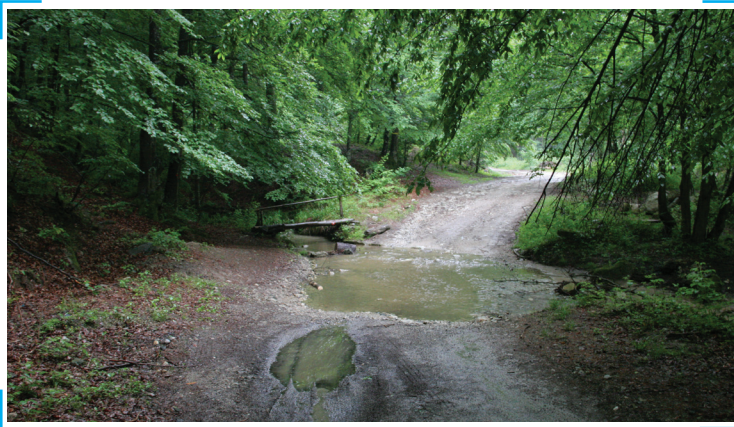
Picture 3: A ford made from concrete or stone should be foreseen at the planning phase of a creek crossing like the one shown above (Photo: Juri Beguš)
