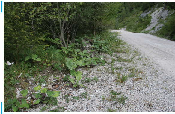
Picture 14: Vegetation on the left side of the picture makes normal grading impossible (Photo: Juri Beguš)
