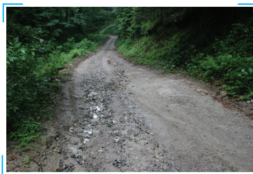
Picture 20: Solutions for the problem in the picture are: removing vegetation, constructing a side ditch, filling the carriageway with gravel, grading the carriageway, and shaping the crown profile, compaction (Photo: Juri Beguš)
