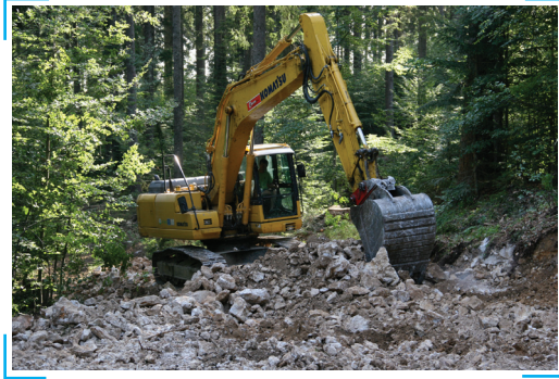
Picture 24: Nowadays excavators are one of the most appropriate pieces of equipment for maintenance of forest roads (Photo: Juri Beguš)
