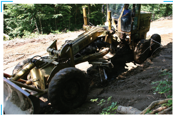
Picture 16: Shaping of side ditch with grader blade (Photo: Juri Beguš)
