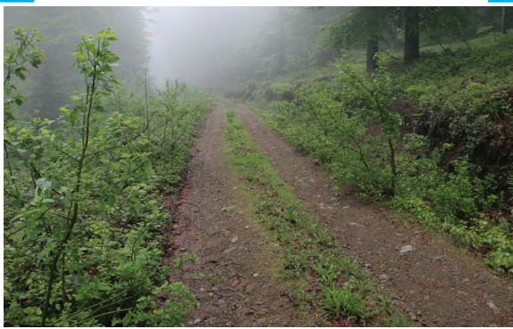
Picture 7: Roadside with inadequate clearing of vegetation (Photo: Juri Beguš)
