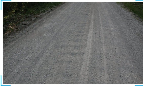
Picture 6: Rolling carriageway can cause damage to vehicles (Photo: Juri Beguš)
