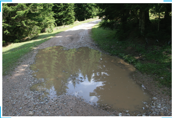
Picture 19: Pothole can cause damage to vehicles (Photo: Juri Beguš)
