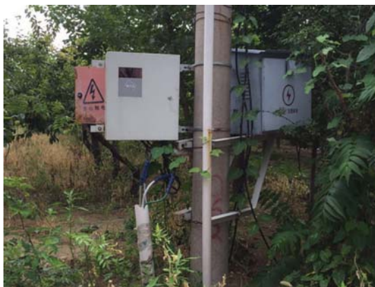
Figure J5: Outdoor Open-type and Simple Well-type IC Card Control Box
