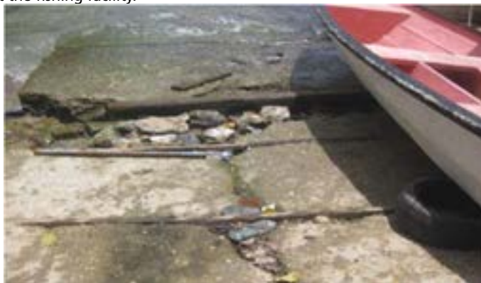
Figure 1: Defective ramp at the Blanchisseuse Fishing Facility.
