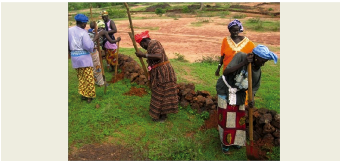
Figure 5. Improving soil health trough constructing natural stone walls
