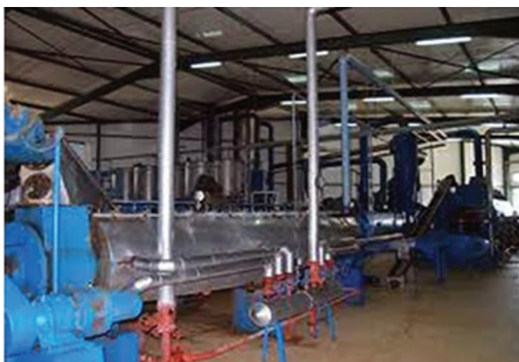
FIGURE 6.5 Photo of a fish meal factory in Nouadhibou
