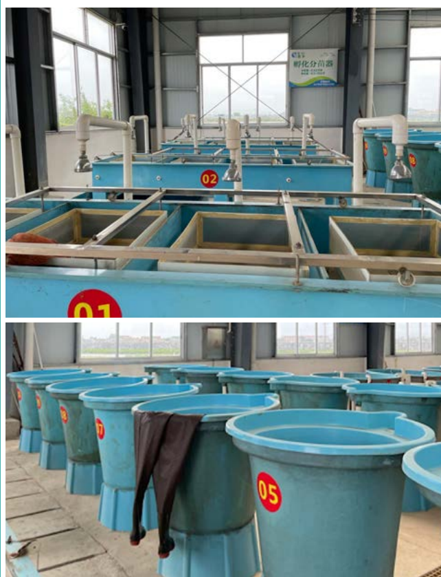
FIGURE 6.10 Construction of hatcheries with the water recirculating system in the aquapark
