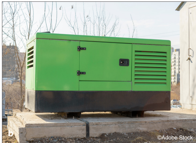
Figure 15.3. a and b Backup generators may be necessary for continuous power supply (images courtesy of Adobe Stock)
