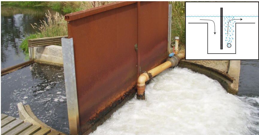
Figure 2.10 Aeration well system using the air-lift principle
