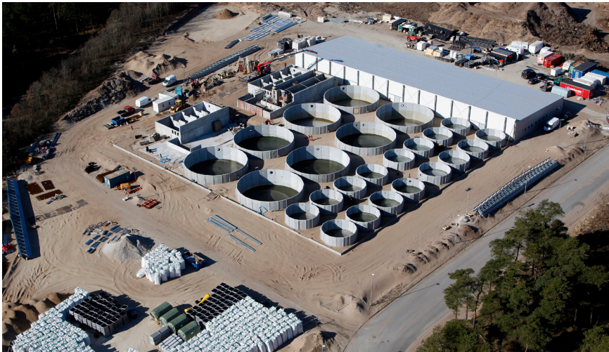
This 2 000 tonnes salmon farm in Hirtshals, Denmark was built in 2013. The system is based on recirculation technology and is covered by a building to control temperature and for high biosecurity. Salmon are grown from eggs to around 4–5 kg size in 2 years in large tanks of almost 1 000 m 3 each. The white bigbags in the foreground are packed with biomedica ready to be filled into the biofilter chambers. Source: Axel Sjøgaard/AKVA group.
