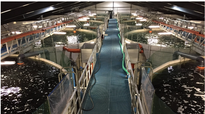
Figure 1.1 An indoor recirculation system
