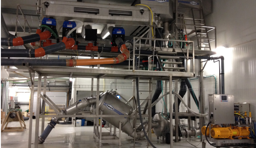
Figure 5.10 The vacuum pump below pumps live fish from a fish tank to the grader above
