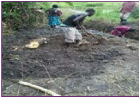
Repairing a drainage canal during pond renovation, Uganda, ©FAO/Mulonda Boniface.
