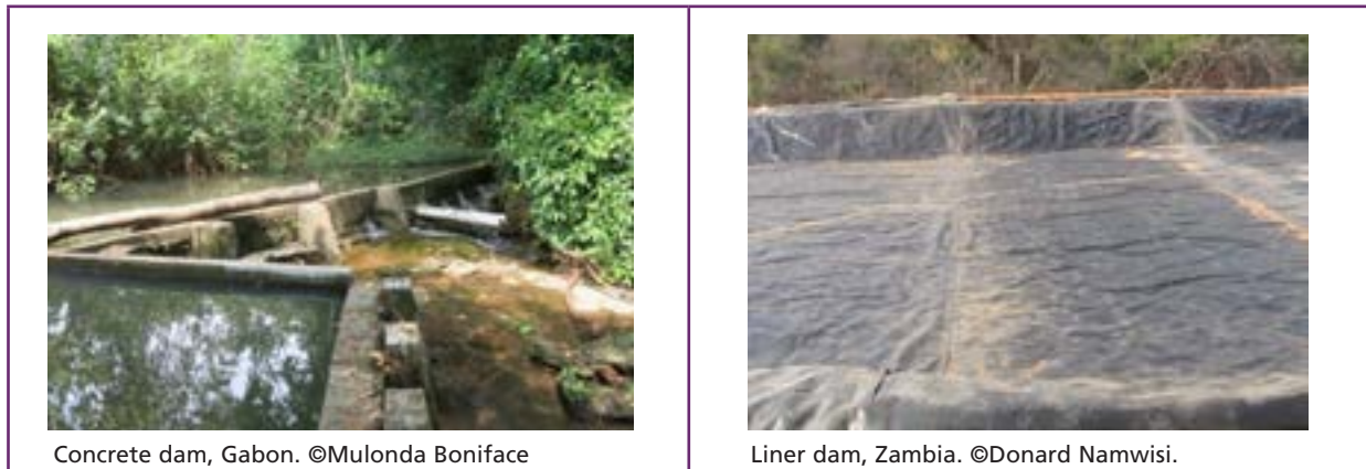
Concrete dam, Gabon. ©Mulonda Boniface
