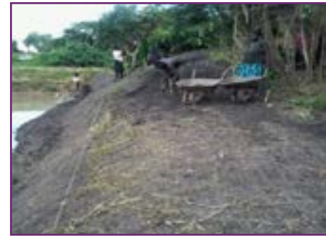
Shaving a dyke during renovation, Uganda, ©FAO/Mulonda Boniface.
