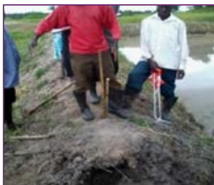
Dyke demarcation/staking out for renovation, Uganda, ©FAO/Mulonda Boniface.
