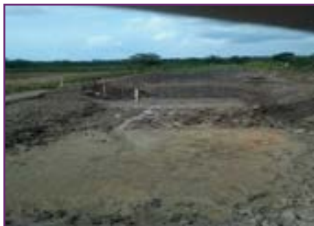
During renovation, leave open the drainage point to dry the pond bottom, Uganda, ©FAO/Owan Simon.
