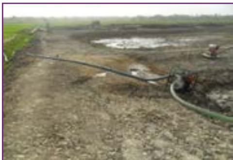
Mechanical soil compacting and drainage of excessive water, Guinea-Bissau, ©FAO/Issa Barry.
