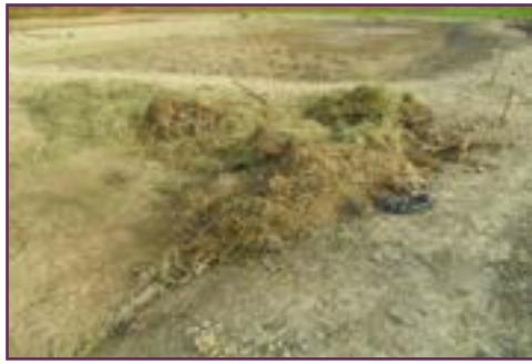
Preparing a pond renovation by cleaning the site, Guinea-Bissau, ©FAO/Mulonda Boniface.
