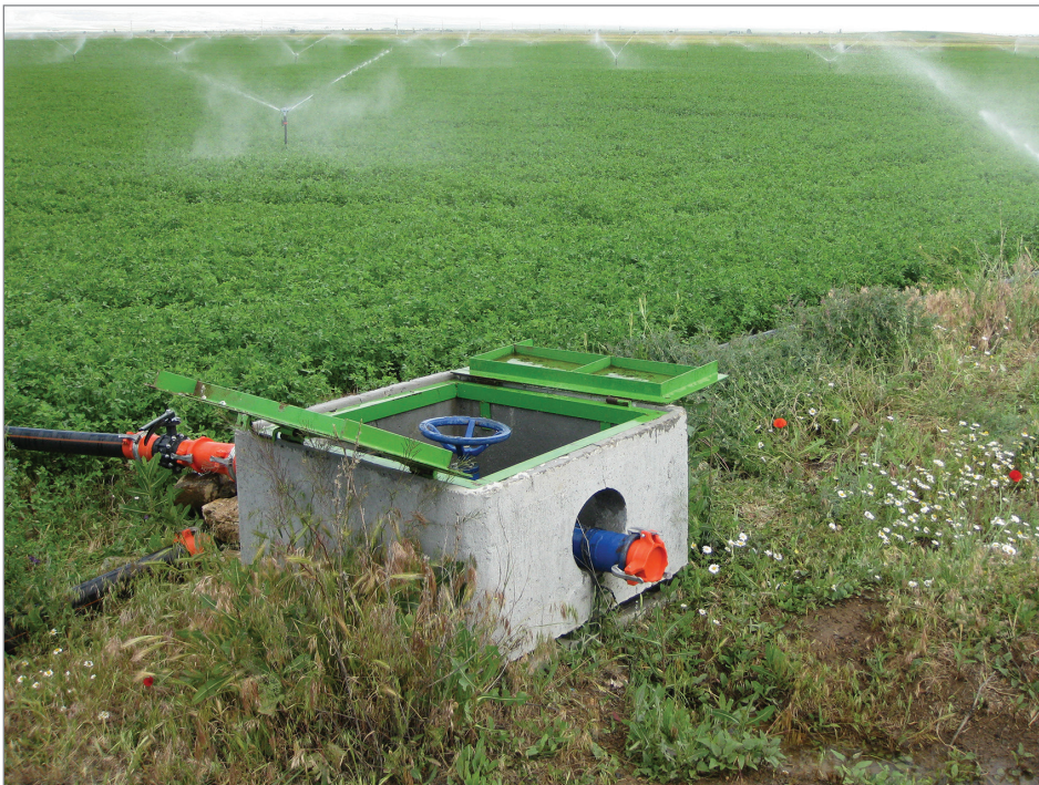
Rehabilitated irrigation system in land consolidation project in Cuimra, Konya province, Turkey (2014). © FAO.
