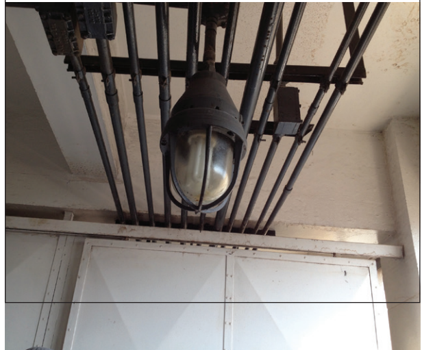
FIGURE 13 Light well protected
