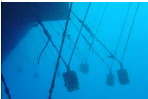
PLATE 31 Concrete sinkers – correct installation
