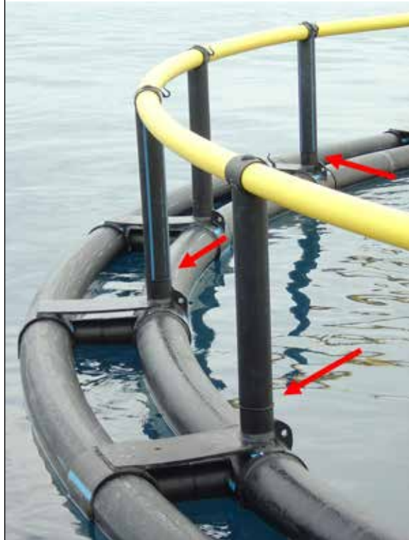
PLATE 24 HDPE brackets made with welded HDPE pipes, mounted on a cage. Note the butt welds on the stanchion (red arrows), which are less robust
