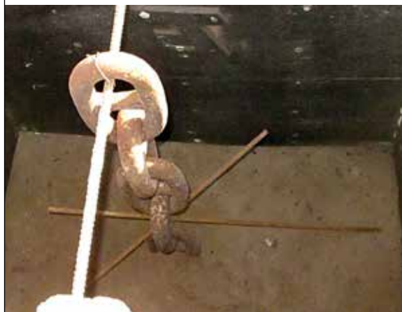
PLATE 6 Detail of the stud link chain used in the wooden form. Note the two iron bars added on the lower link
