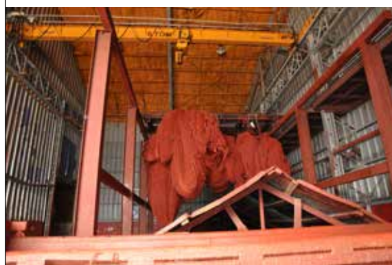
PLATE 77 A net treatment plant
