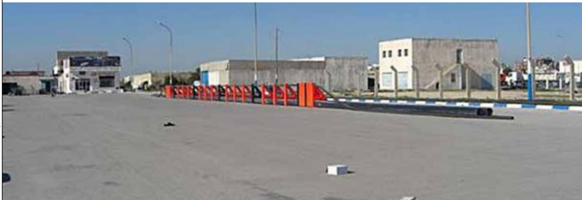
PLATE 41 The two main pipes after their construction. The pipes have already been inserted through the brackets, which are distributed along half of the pipe length. The handrail has been inserted as well
