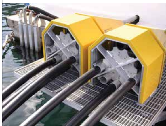
PLATE 112 Detail of a centralized feed system. Visible are two feed distribution units from which several HDPE pipes convey the feed to the cages
