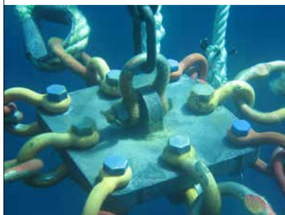
PLATE 14 Corner plate, eight holes. Four are used to connect the main mooring lines; four are used to connect paired mooring bridles for the cages
