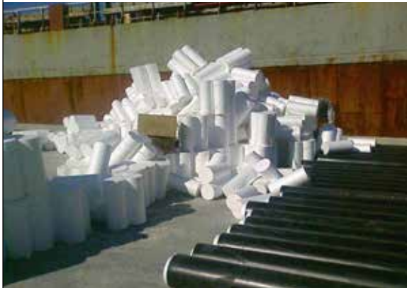
PLATE 40 Polystyrene cylinders are inserted into the pipes
