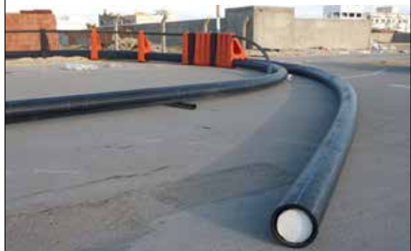
PLATE 43 Detail of the pipe end: the polystyrene cylinder is visible. Also the handrail is strung through the upper hole of the stanchions
