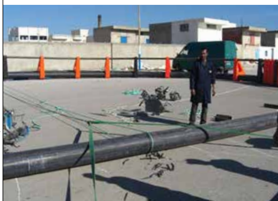
PLATE 42 Pipes are bent into a complete circle
