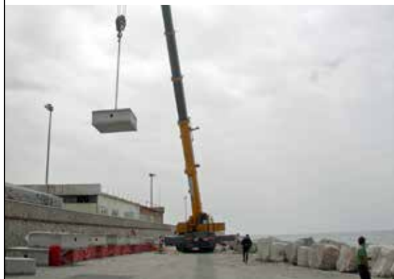
PLATE 8 Concrete block deployment. The concrete block is lifted into place using the boat's crane or lift bags
