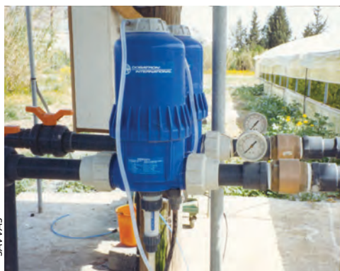
Plate 3 Supply of nutrients through the irrigation system using a system of dosing pumps to inject stock solutions to the irrigation pipe
