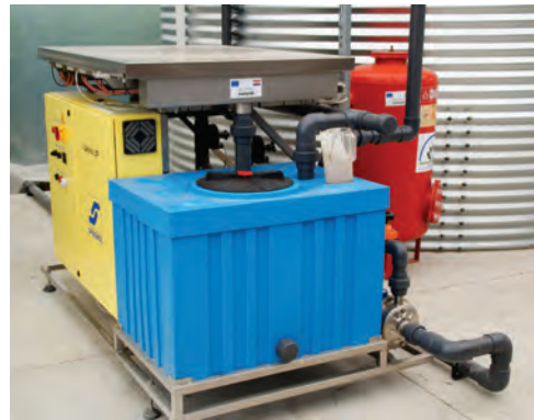
Plate 4 Filtration and UV sterilization unit
