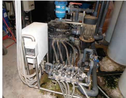
Plate 8 Preparation of nutrient solution for soilless-cultivated plants using an automatic fertigation head to control EC and pH of outgoing solution
